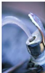
Water flowing through the aspirator created suction that drew body fluids through a hose and into the funeral home's water supply. The combination of low water pressure and suction created by the aspirator caused body fluids to be back-siphoned into the funeral home's water supply and threatened the public water system.
