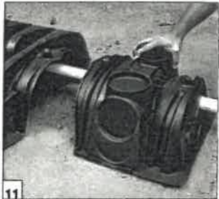
Lateral pipe through end cap.
