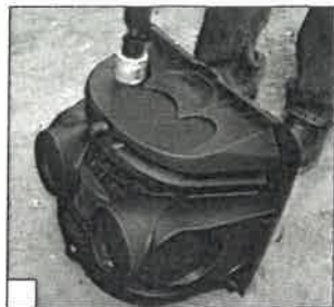
Drill pressure pipe hole.
