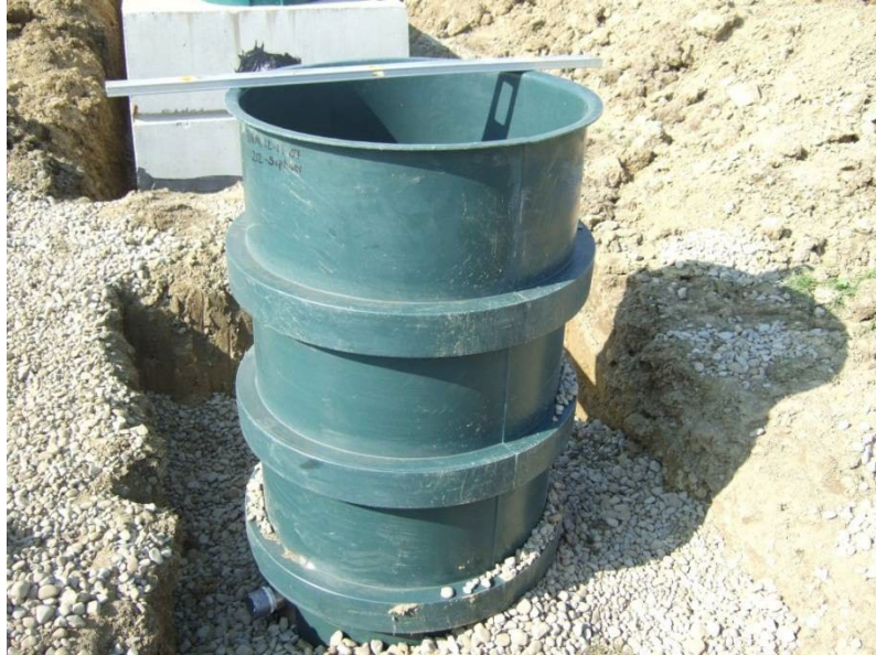
Figure 5. Dosing siphon - external view
