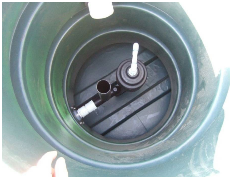
Figure 6. Dosing siphon - internal view
